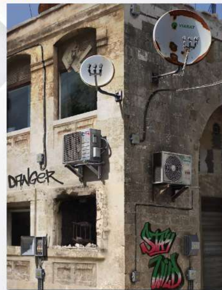
35638 AIR CONDITIONERS &amp; SATELLITE DISHS
